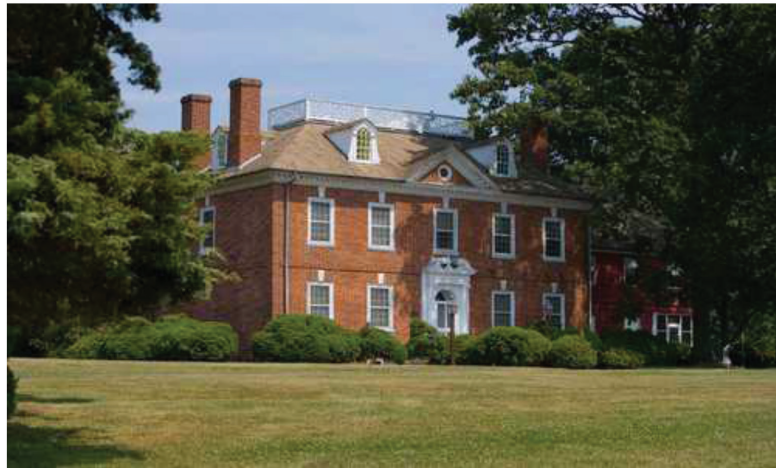
Mount Harmon Plantation originated as a land grant of 350 acres to Godfrey Harmon by Caecilium Calvert the second Lord Baltimore, in 1651. It prospered as a tobacco plantation during the 17th and 18th centuries, growing and exporting tobacco to the British Isles.
